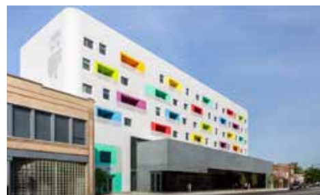
Chicago, IL branch library mixed use project: 16,000 sq ft library and 44 units of affordable senior apartments
