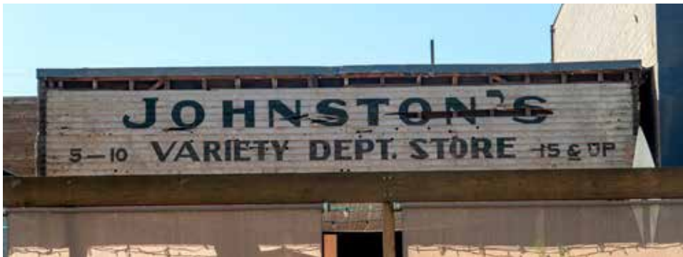
Historic Sign Uncovered at 4628 Park Blvd. in University Heights
