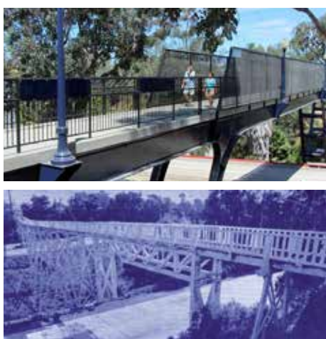
Vermont St. Bridge circa 1976
