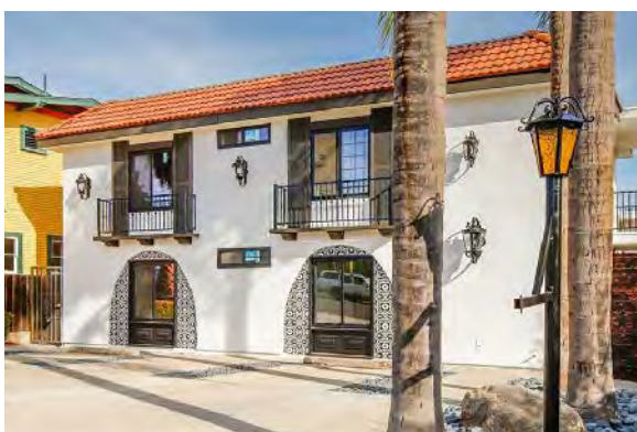
3233 Herman Ave. 8 units. Built in 1972. Renovated in 2018.
