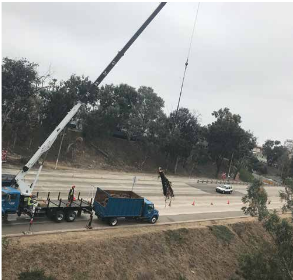
Clean out in process at Camelot Canyon near 163 freeway on ramp.
