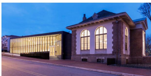
New York Public Library, Stapleton Branch, Staten Island. Example of blending new and existing construction together.
