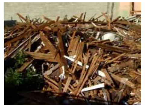
Demolished house, Friday May 29, 2015.
